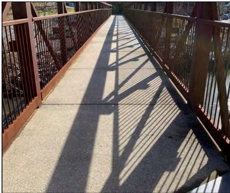
Image 4: Bridge Walking Surface
