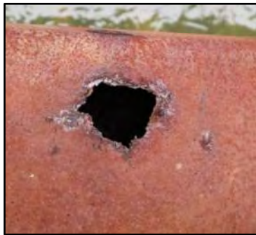
Image 7: Close-up of Holes through Bottom Chord
