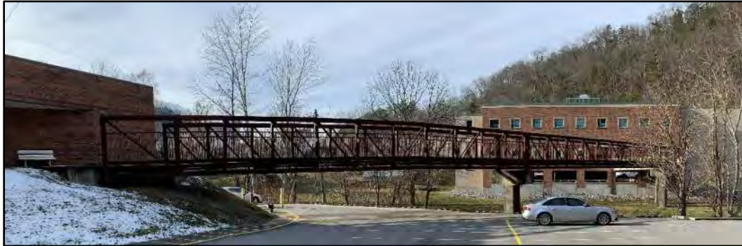
Image 3: Bridge East Elevation
