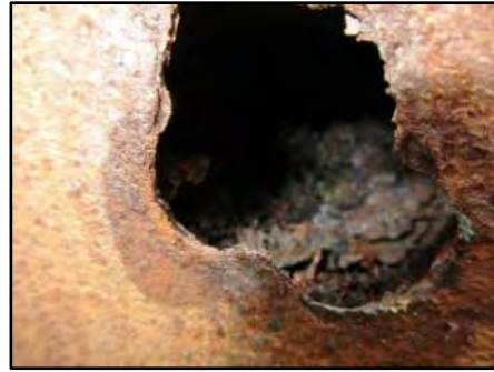
Image 7: Close-up of Holes through Bottom Chord
